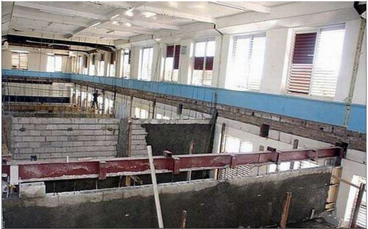
O'Hare Restoration in progress at June,2009
